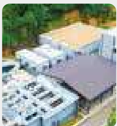
Water and Wastewater Purification
